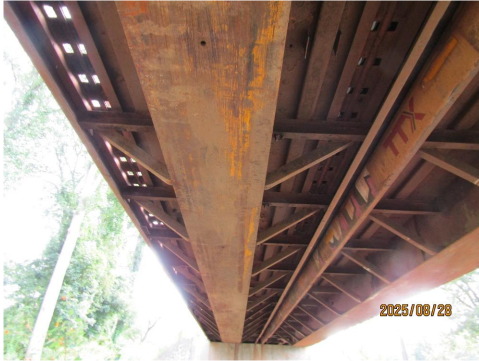
Figure 2: Refurbished railroad flatcar deck structural elements
