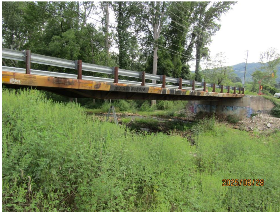
Figure 1: Railcar bridge at Warren Wilson Rd. in Swannanoa, NC
